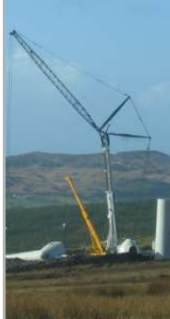
Some wind farm turbine erection
