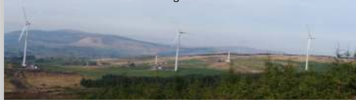
Bawnmore wind farm during turbine erection
