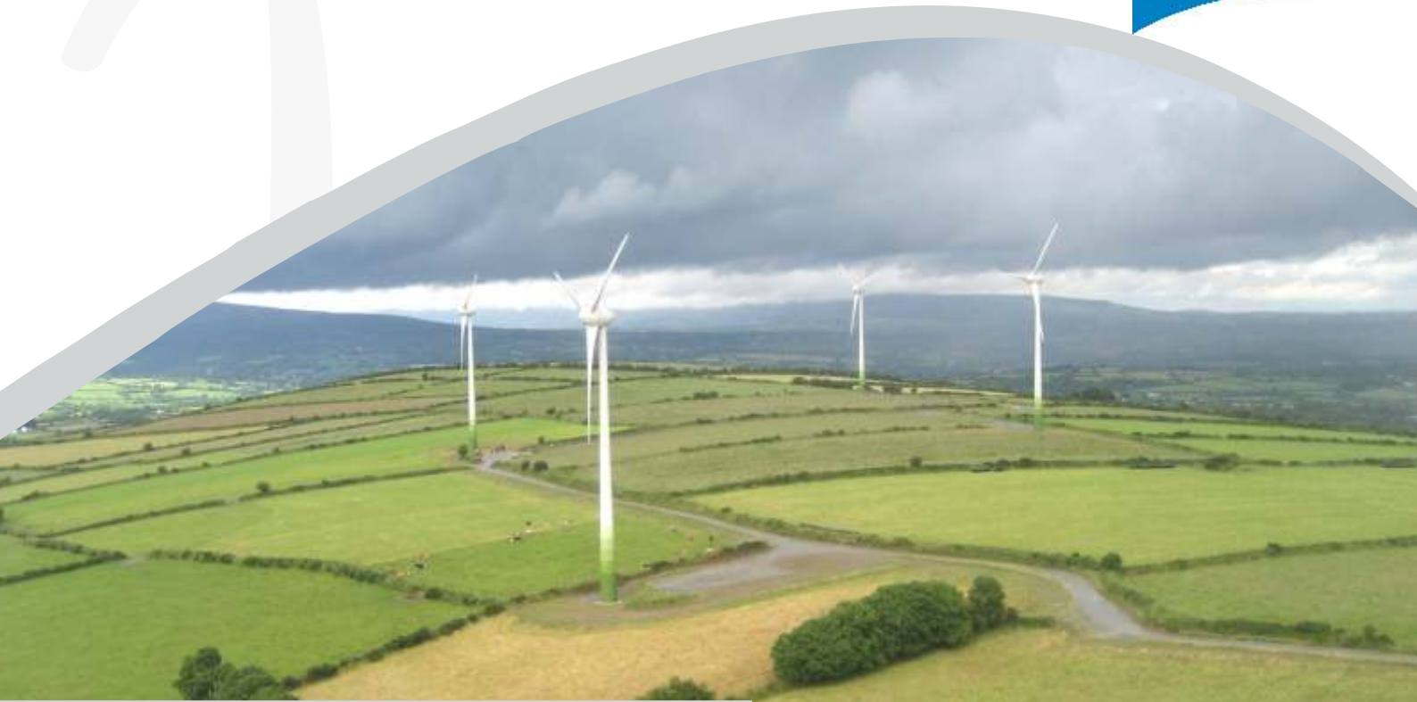
Rahora wind farm during final commissioning
