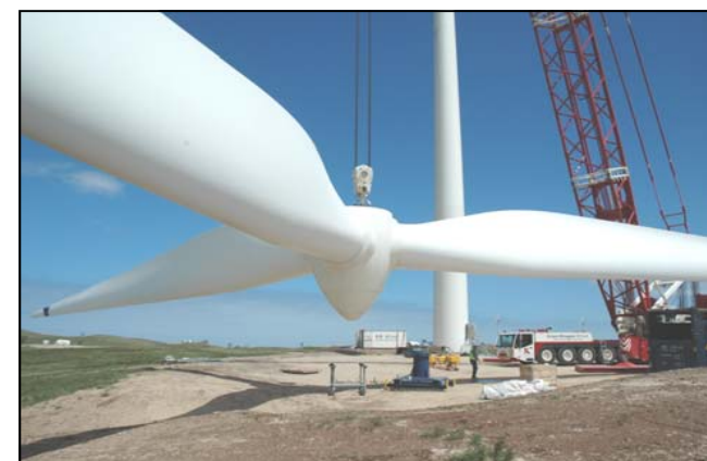
Rotor installation
