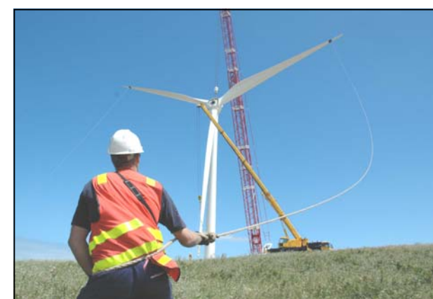
Rotor installation
